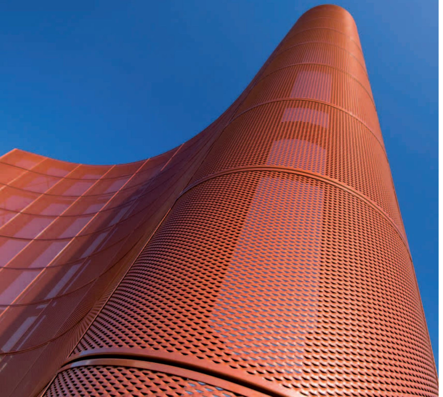
Detailed elevation showing the joints between the two wings of the cladding.
